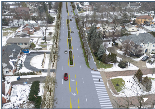
Renderings of the 5 Lane Option (with a shared use path on one side); see pages 20-25 for more information.
